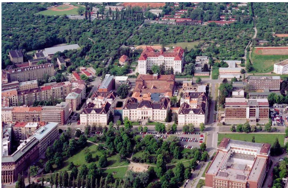
General view on the complex of buildings of the Faculty of Civil Engineering BUT, Brno
